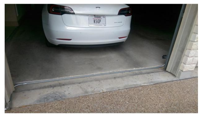
Another view showing the routing of the conduit to the inverter box and 240 volt outlet.
