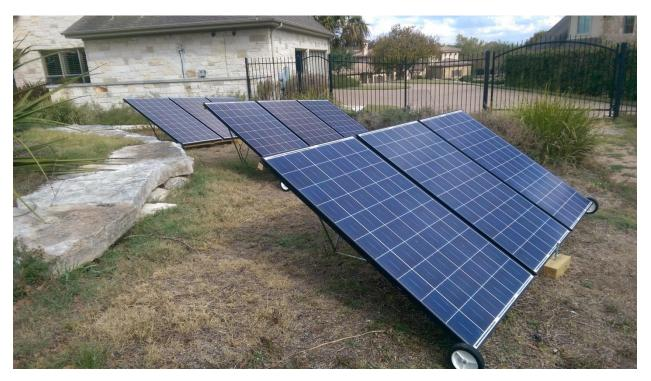
The panels are on wheels for manual tracking of the sun and pivot around a ground rod at the base. Clamps at the base and an anchor to ground prevents the panels from blowing over in high winds.
