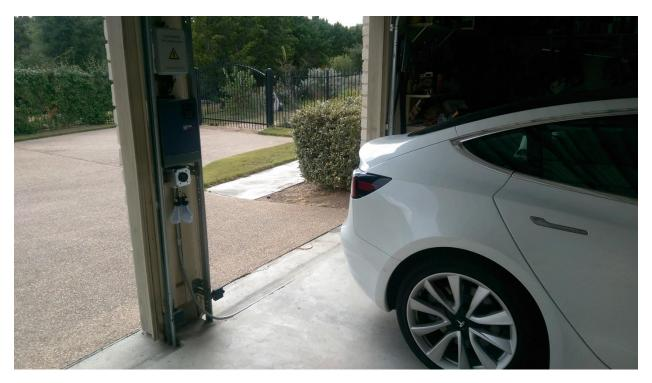
The PV combiner box has a switch and a surge protector. The DC current from the panels is about 330 volts at 8 amps full sun. Wiring is enclosed for safety and NEC standards.
