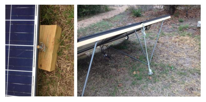
The metal tubes are triangular shaped and give the panels rigidity. The angle is set to slightly over 30 degrees elevation to maximize the sun angle for the year. The south facing panels are spaced in the back yard to receive maximum sunshine considering the surrounding fences and trees. The panels can be rotated during the day for morning and evening collecting more energy than if left just facing south.
