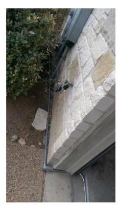
Here is the detail how the conduit runs along the garage opening. The garage door does not touch the conduit at any location.
